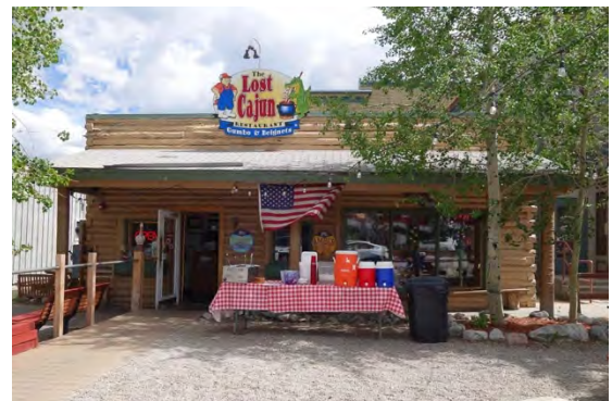
204 Main St • 5ST.1759 • Lost Cajun 1952 • This log building with a low false front characterizes the type of construction that was typical in the mid-century as tourism began to become a trend in this area.
